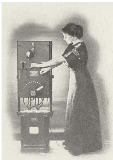
An early home charging station Click on the Photo for the Link
