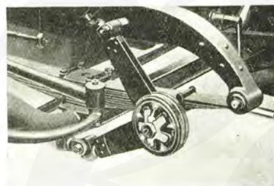
Fig. 34. Showing Shock Absorbers in position and Adjustment Indicator.
