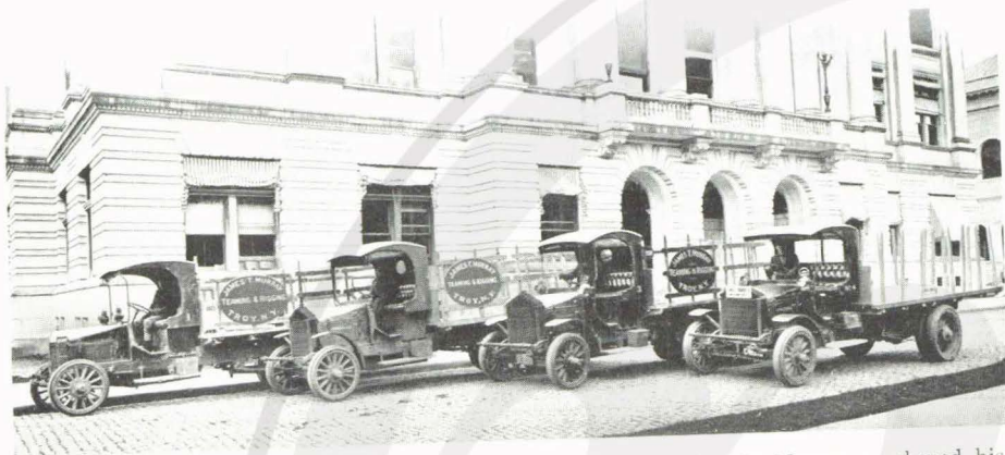
James T. Murray, Rigging and Heavy Trucking, Troy, N. Y. Mr. Murray purchased his first 5-ton Pierce-Arrow truck in August, 1911. Subsequent orders have increased his fleet to five. These trucks are used to perform very varied duties, such as towing canal boats, hoisting stacks, delivering coal and hauling in connection with road building.
