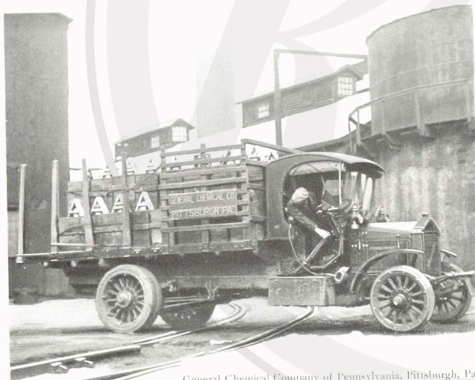
General Chemical Company, Laurel Hill, L. I. Interchangeable bodies
