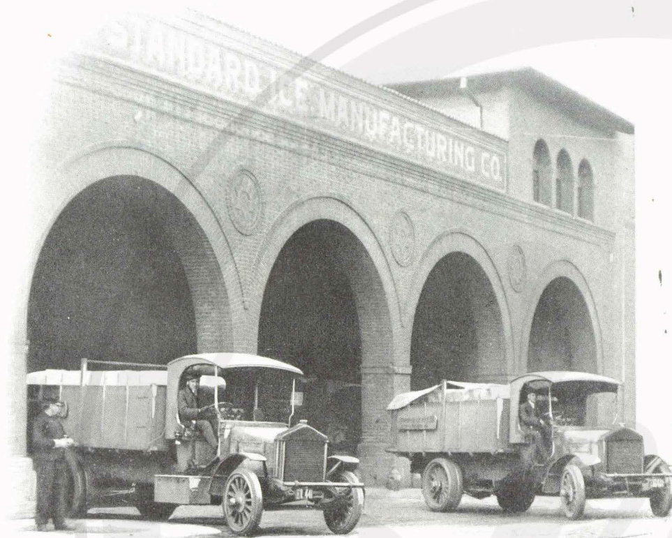
Standard Ice Manufacturing Company, Philadelphia, Pa. Using three 5-ton Pierce-Arrow trucks and hauling an average of over 50 tons per day on runs that average three miles out from the manufacturing plant to the distributing stations.
