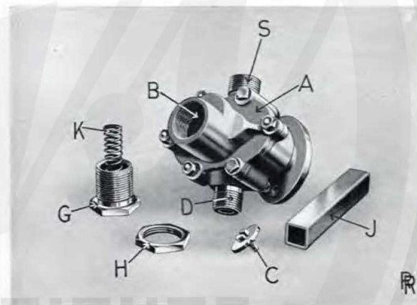
FIG. 6. ENGINE OIL PUMP DISMANTLED.
