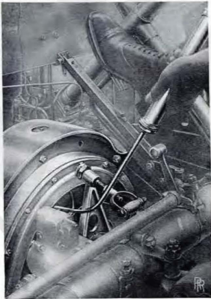
FIG. 7. OILING CLUTCH SURFACE.
