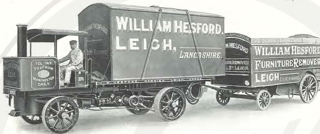
Class "H" Chassis with 14ft. 6in. platform. Carrying Lift Van and drawing Pantechon. (For Lift-off Van Bodies see page 46.)
