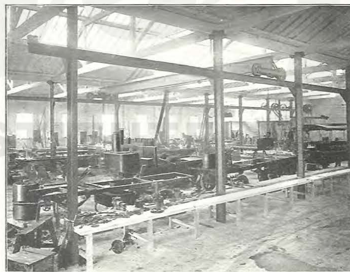
General View of Repairs Bay.
