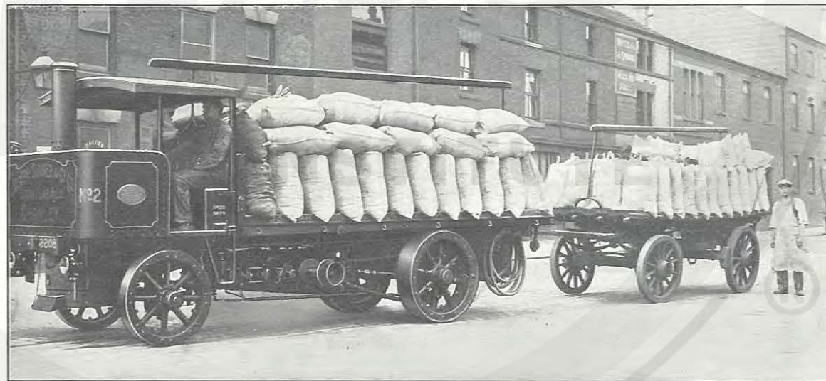
Standard 6-Ton WAGON and TRAILER. Showing Winding Drum.
