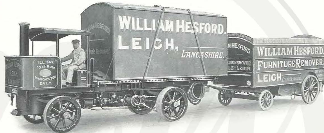
Standard 5-Ton WAGON with 13-ft. 6-in. Platform. Carrying Lift Van and drawing Pantechicon.
