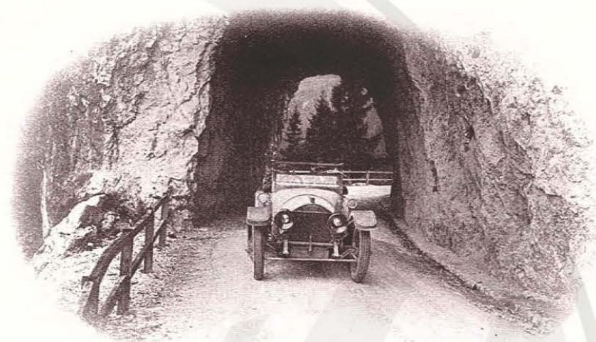
One of the Tunnels of the Ampezzo Pass.
