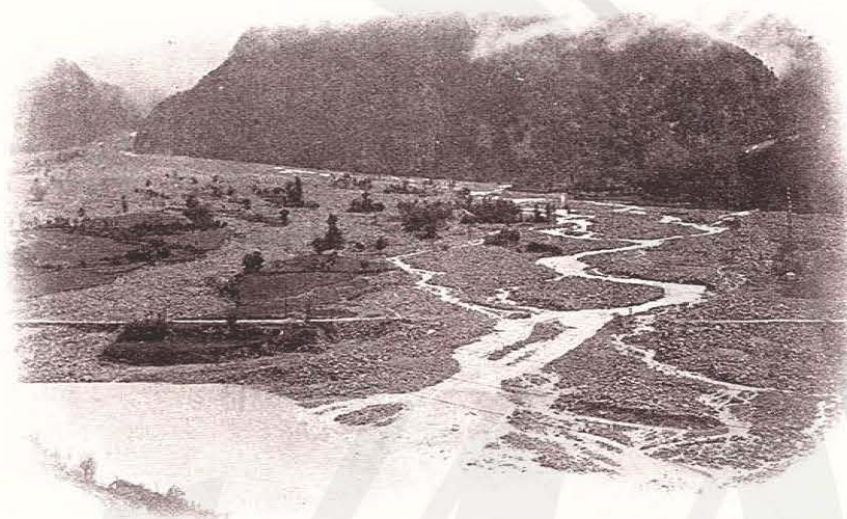
The direct road to the Aprica Pass, washed away owing to an Avalanche.
