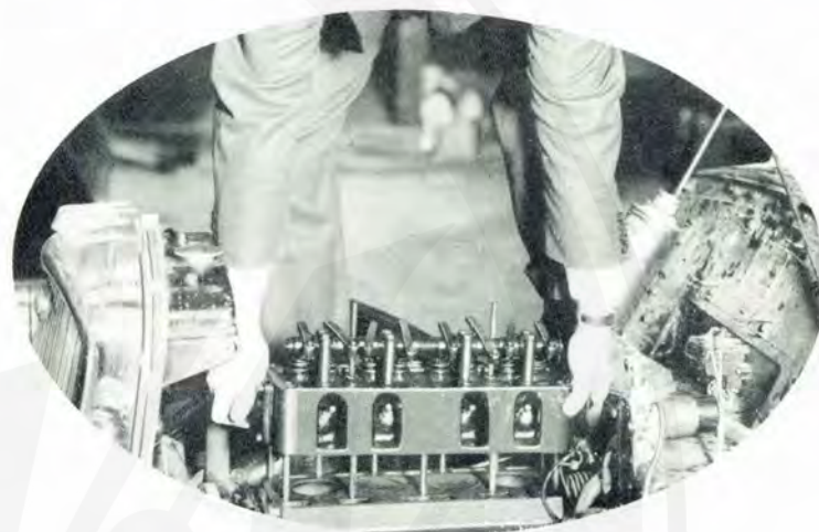
Withdrawing the cylinder head.
