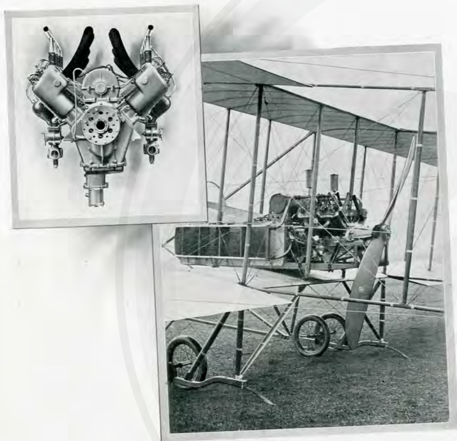
Farman biplane fitted with Sunbeam-Coatalen 150 h.p. 8-cylinder aircraft engine, "Crusader" type.
