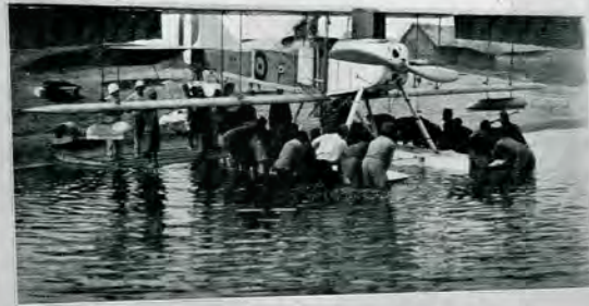
Sunbeam engined seaplane at Lake Tanganyika. This was the first seaplane ever flown over this Lake, which is situated 2,670 feet above sea level. It was fitted with 150 h.p. 8-cylinder Sunbeam-Coatalen engine, and carried out many excellent flights, the high altitude calling for a very high engine efficiency. An interesting incident in the career of this seaplane was the bombing of the German gunboat "Graf von Gotzen" at Kigoma.
