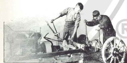
After assembling, Chalmers axles are tested under load in a chassis.
