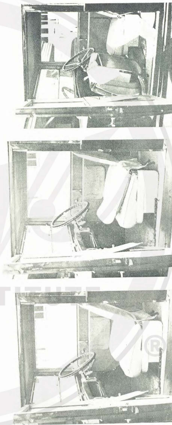
FIGS. 9, 10, 11.—THREE VIEWS OF THE ADJUSTABLE FRONT SEATS OF THE 11 H.P. "STANDARD" SALOON ("PICCADILLY" MODEL). The rear seat is shown in three positions, viz.: (a) ready for use, (e) with the back-rest hinged forward to permit access to the rear compartment, and (3) with the seat as a whole hinged forward to provide an exceptionally roomy entrance to the rear compartment.
